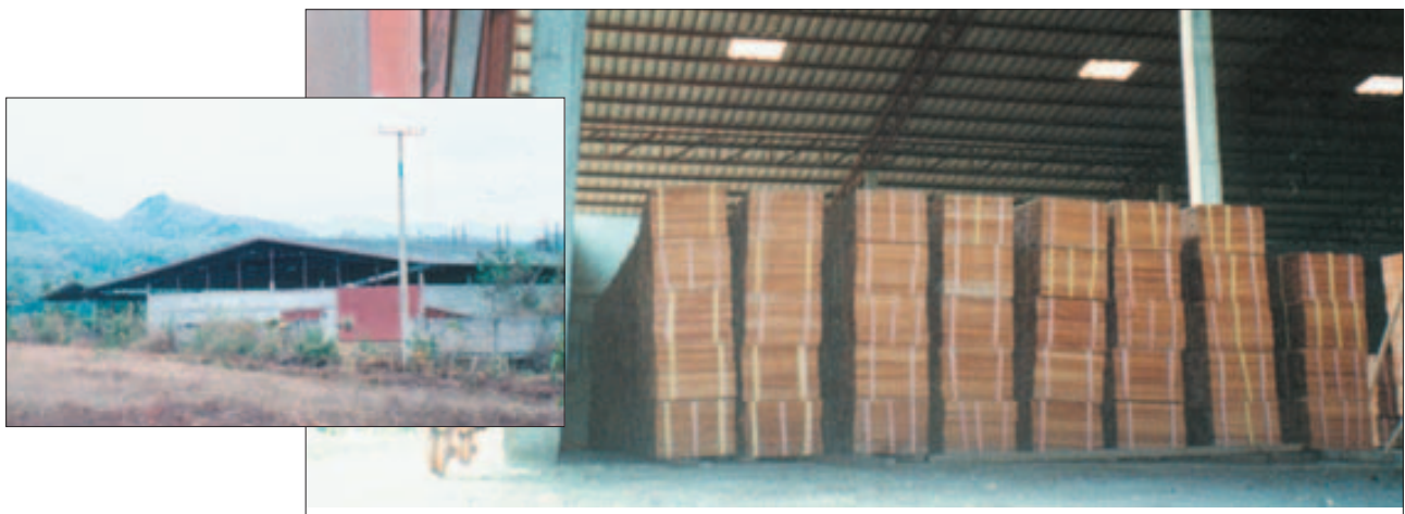
According to locals the sawmill had been closed for 4 years. Upon closer inspection it was found to be storing over 100m 3 of processed teak, Mae Hong Son Province, Thailand; 2001.
