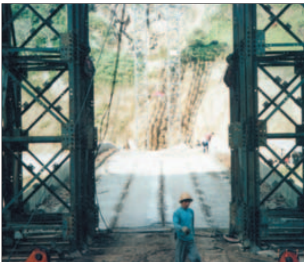
The construction of the bridge at La Cholo.
