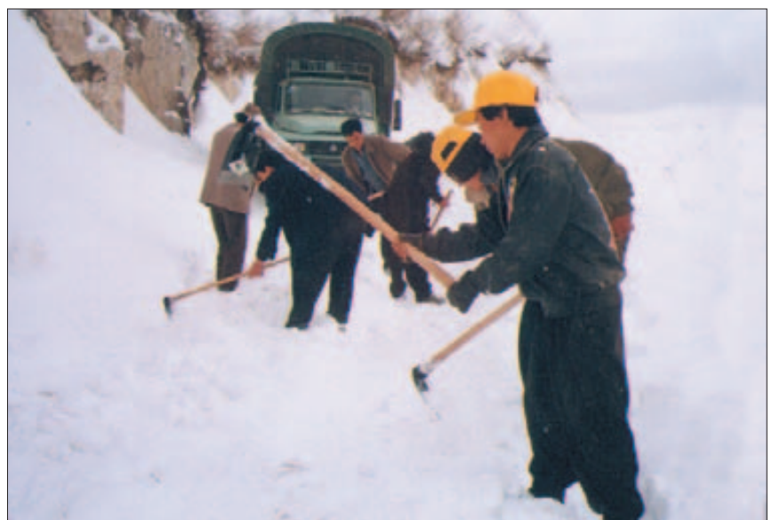
Road leading from China into the N'Mai Hku project area during the winter.
