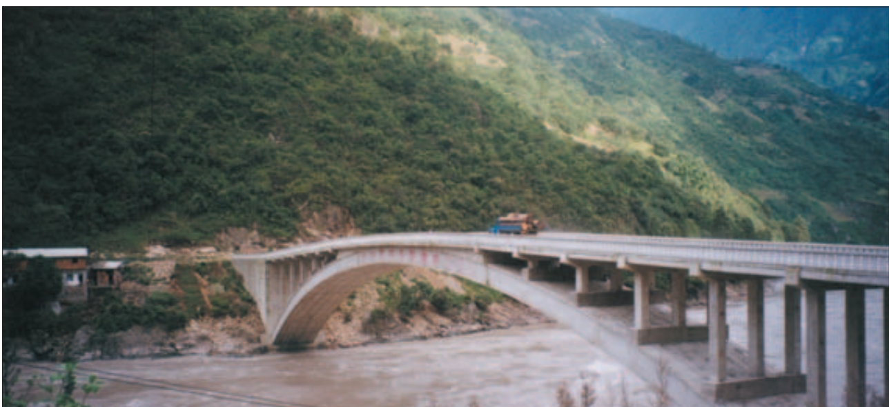
A Chinese truck carrying timber from the N’Mai Hku area across the new La Cholo bridge built to open up Kachin State for exploitation of timber and minerals; 2001. Translation of the words on bridge: “Repair a humble bridge, walk on the road to prosperity.”
