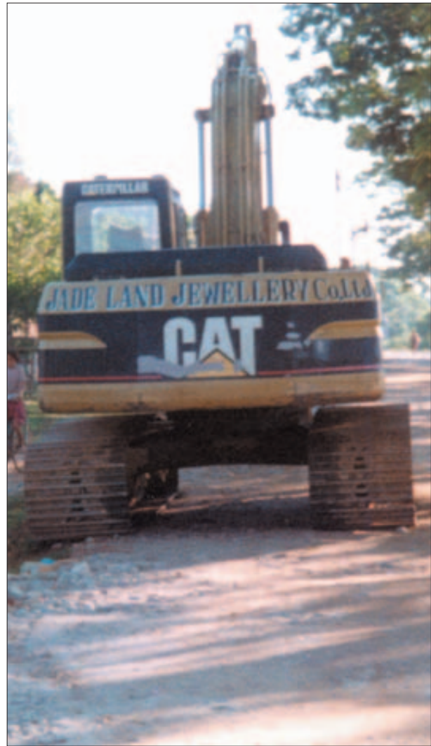
Jade Land machinery being used to improve the road from Myitkyina.
